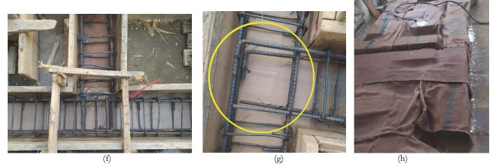
Figure 5: BCJs casting steps. a) BCJ dimensions; b) BCJ separated areas; c) Formwork and steel cages; d) Casting the whole formwork; e) Separation of the casting of the connection; f) condensing of stirrups in the critical lengths, g) sample without stirrups in the joint, h) Samples treatment.
