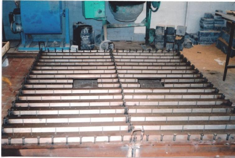
Figure 9: Welded shear studs arrangement along steel beams and sheet ribs; (M3).
