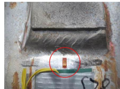
(a) Strain gauge measuring point
