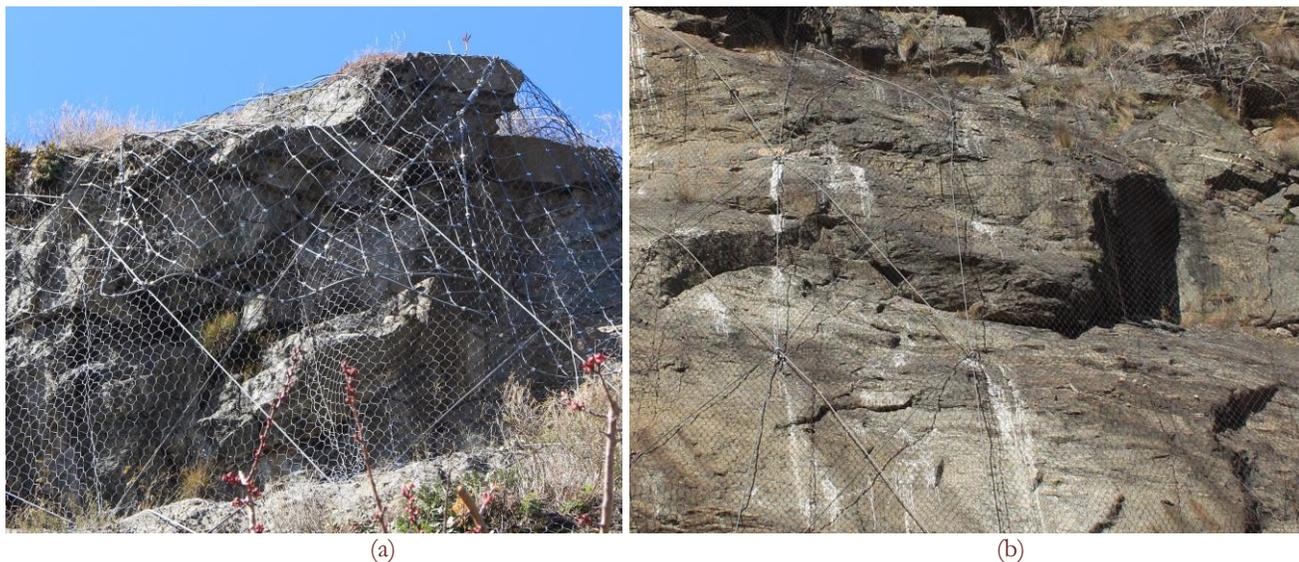
Figure 6: In (a) two mesh types are adopted; in (b) the simple and the reinforced drapery systems are adjacent in the same site.
