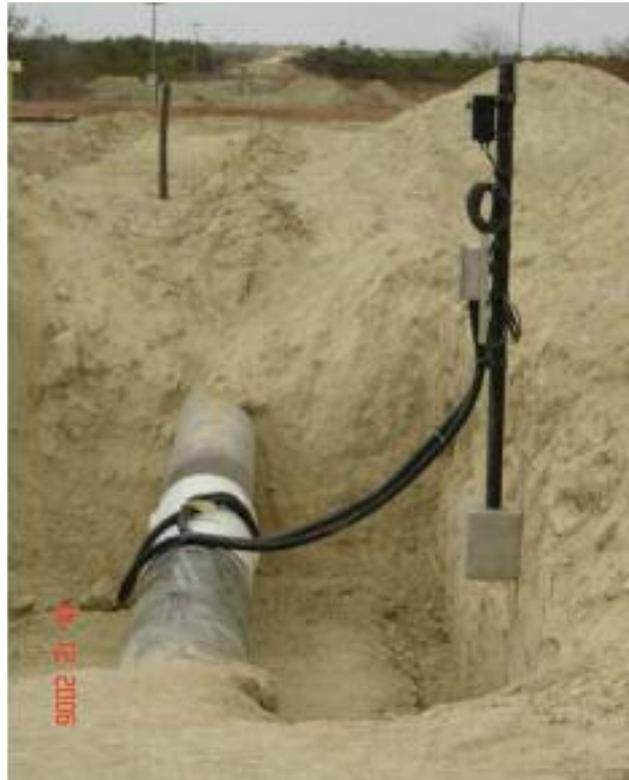
**FIG. 3** *An off-line electric field signature system on an underground pipeline in Brazil. Cable from the instrumented pipe section is pulled to junction boxes for connection with the portable instrument for data collection. After installation, the pipe will be covered by soil, and only the connection post will remain visible.*
