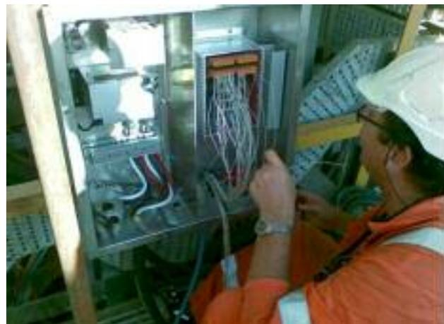
**FIG. 4** *Field cables and termination in an on-line instrument at a refinery.*
