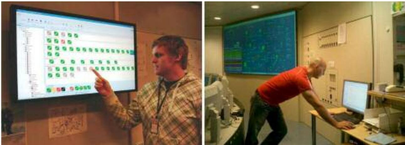
**FIG. 6** Sand Management software installed in the product optimization room and platform control room at the operator. The screen shows the status of each sand probe by colour code.
